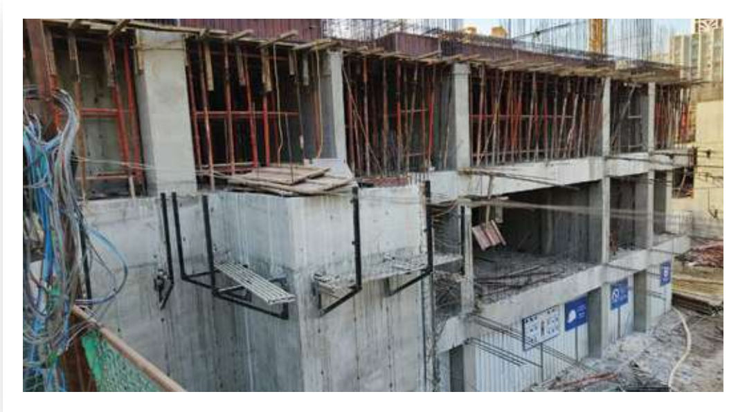
YASHWIN NUOVOCENTRO - 'B' MEZZANINE FLOOR WORK IS IN PROGRESS.
