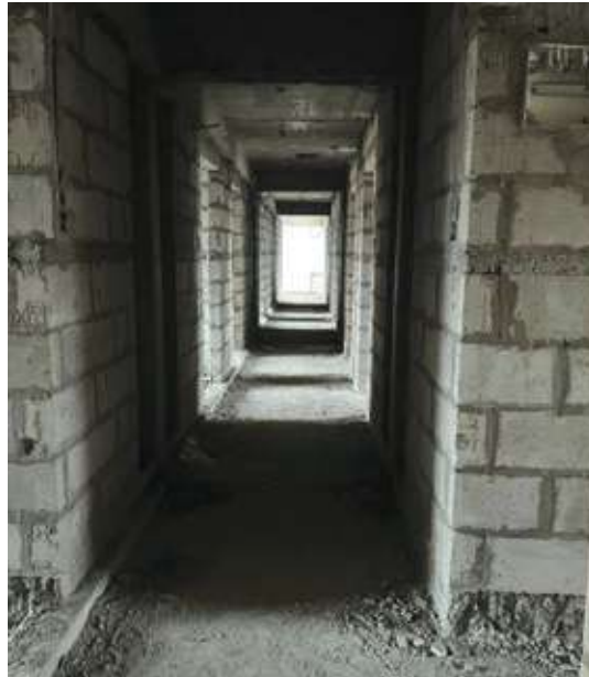
VJ INDILIFE 8TH FLOOR BLOCKWORK IS IN PROGRESS.
