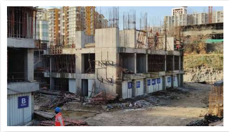
YASHWIN NUOVOCENTRO - 'A' MEZZANINE FLOOR WORK IS IN PROGRESS.
