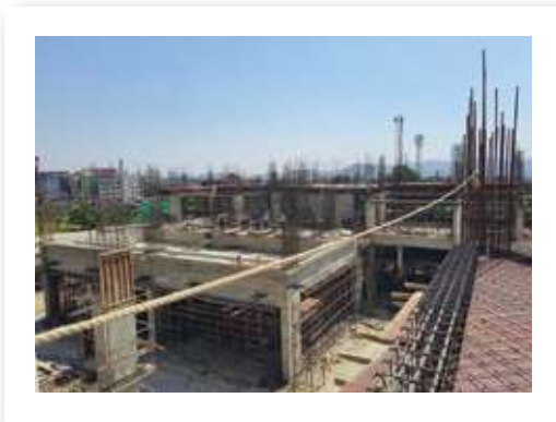
VJ HAPPINESS STREET - RHS MEGA RETAIL SHOP AREA SHUTTERING 60% COMPLETED.
