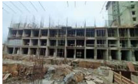
YASHWIN ORIZZONTE - 'D' 3RD FLOOR ALUMINIUM SHUTTERING WORK IS IN PROGRESS.
