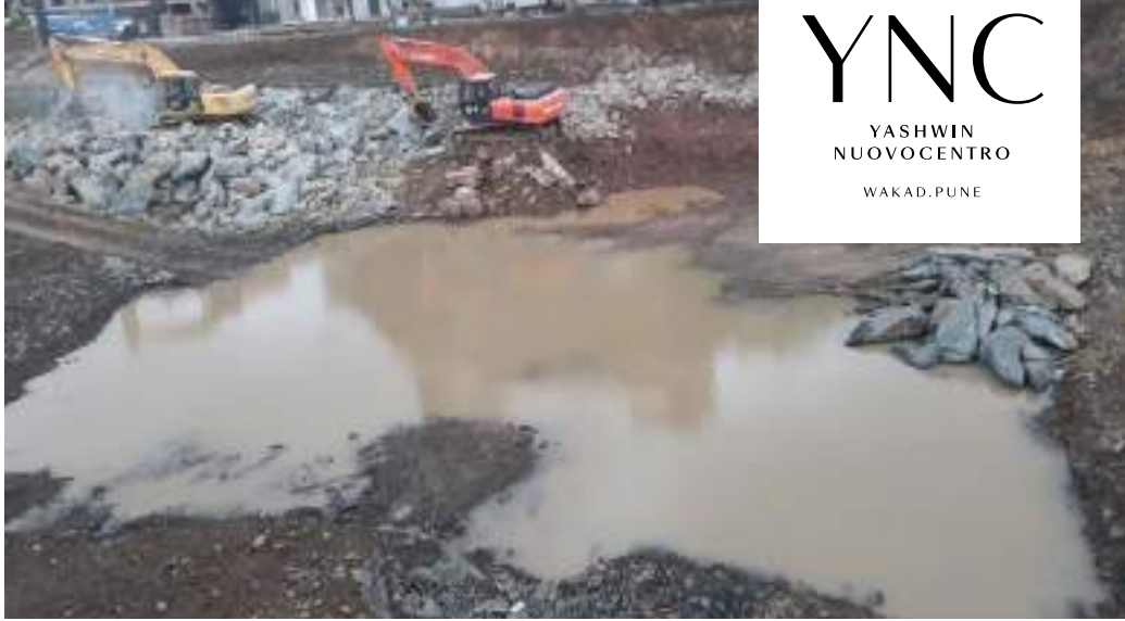
YASHWIN NUOVOCENTRO - 'A' EXCAVATION COMPLETED.
