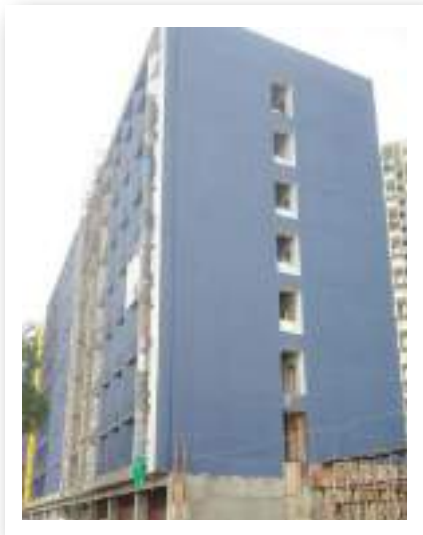
VJ HAPPINESS STREET EXTERNAL PAINTING- 1ST COAT COMPLETED.
