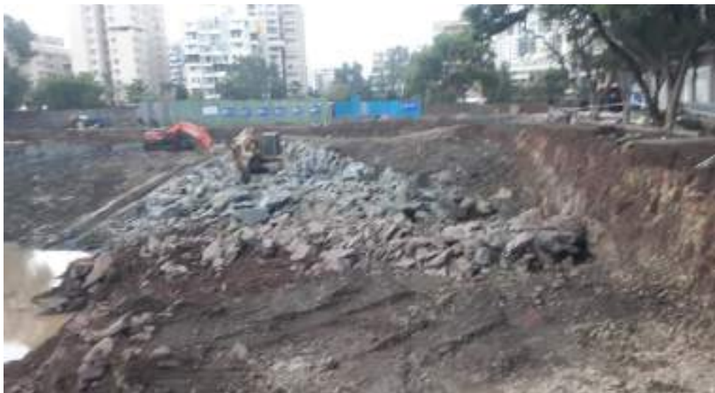
YASHWIN NUOVOCENTRO - 'B' EXCAVATION WORK 40% COMPLETED.
