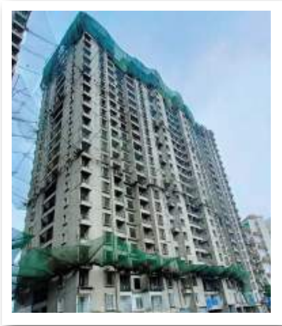
YASHONE INFINITEE - 'D1D2' OHWT, LMR SHUTTERING AND REINFORCEMENT WORK IN PROGRESS.
