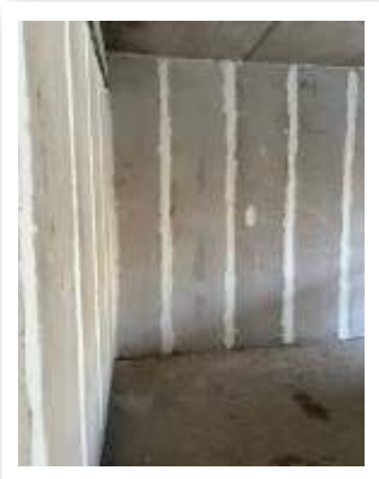
VJ INDILIFE ALC PANEL WORK COMPLETED FOR THE FIRST FLOOR.
