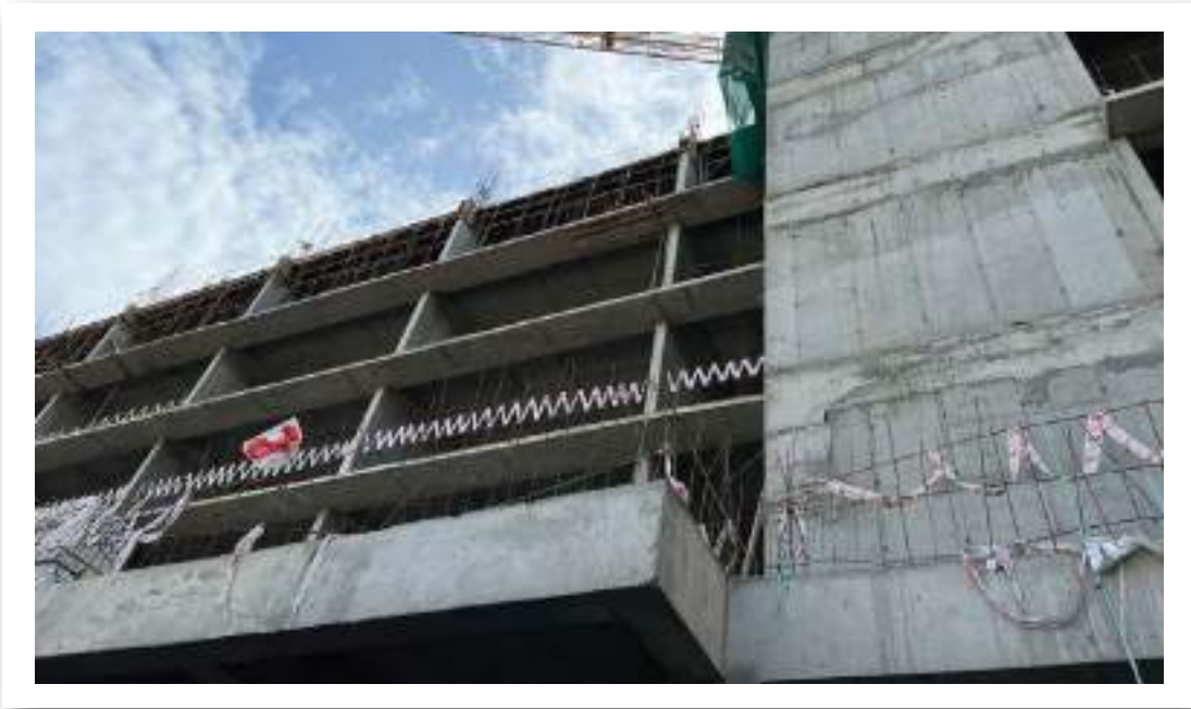
VJ INDILIFE 6TH FLOOR SLAB CASTING COMPLETED.
