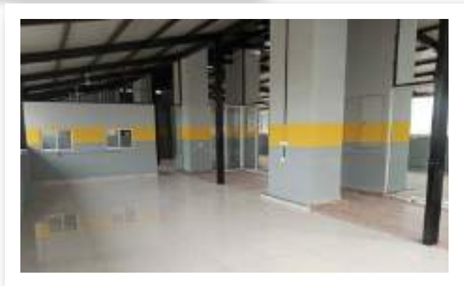
VJ ONE AVENUE TOP TERRACE WORK COMPLETED.
