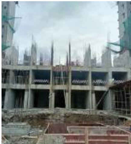
YASHWIN ORIZZONTE - 'C' 2ND FLOOR SHUTTERING WORK IS IN PROGRESS.
