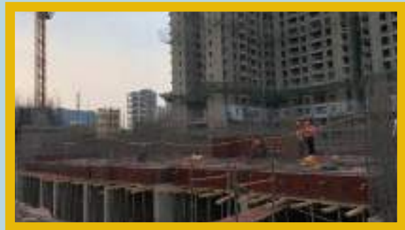
Ground floor slab shuttering Work is in progress
