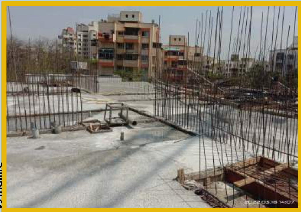
2nd floor slab 1st pour casting done.
