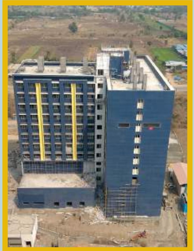
External painting 2nd coat work 90% completed.
