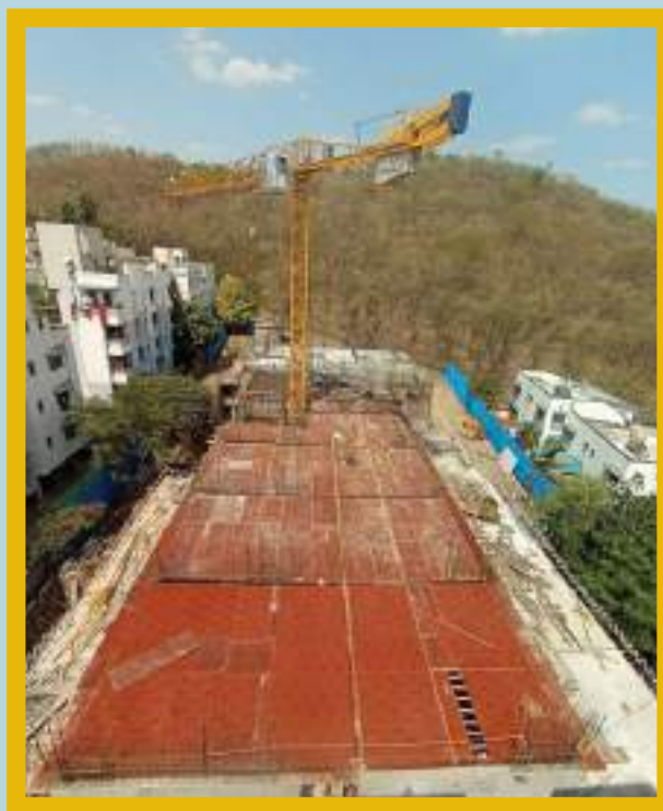
Upper Ground Floor Slab completed.
