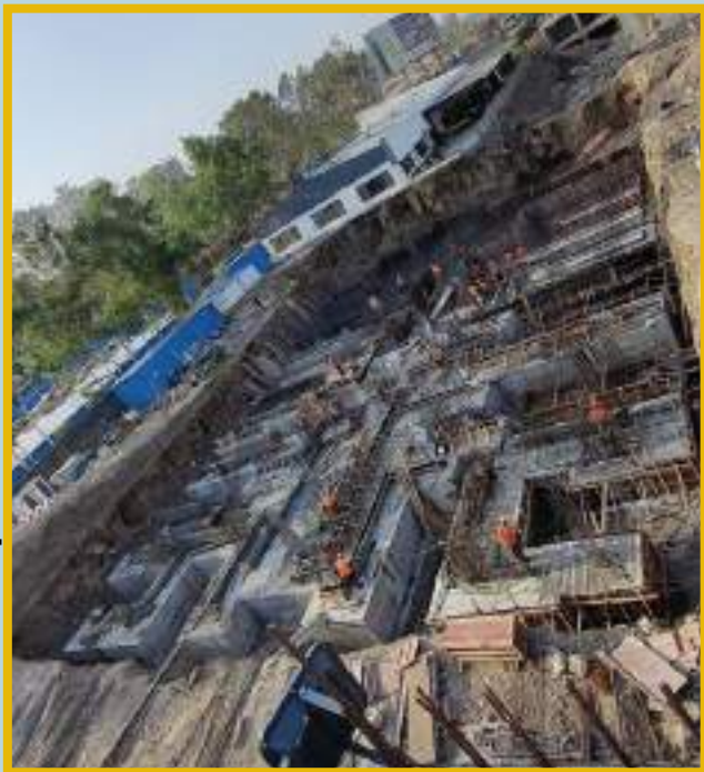
Footing Reinforcement binding & Casting work is in progress.
