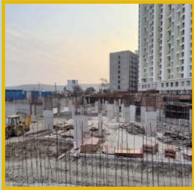
Floor raft work is in progress.
