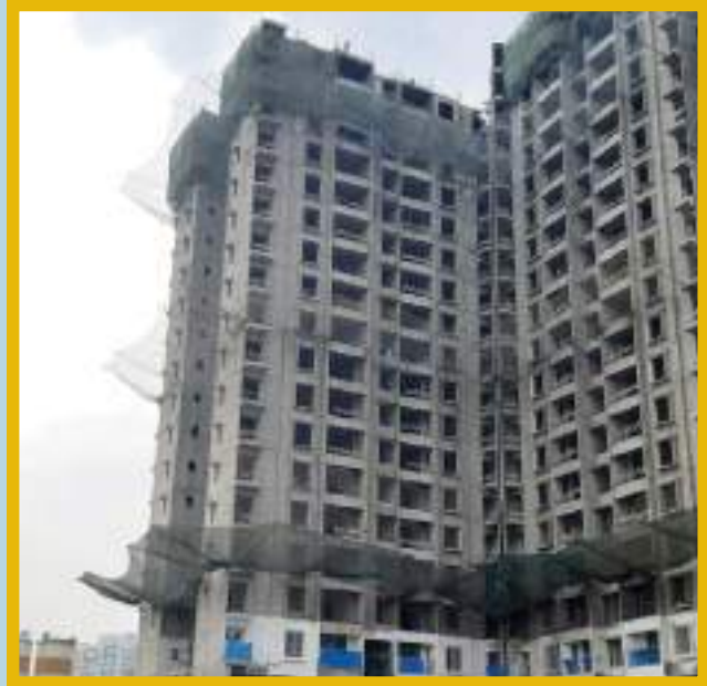
19th floor slab shuttering work is in progress.
