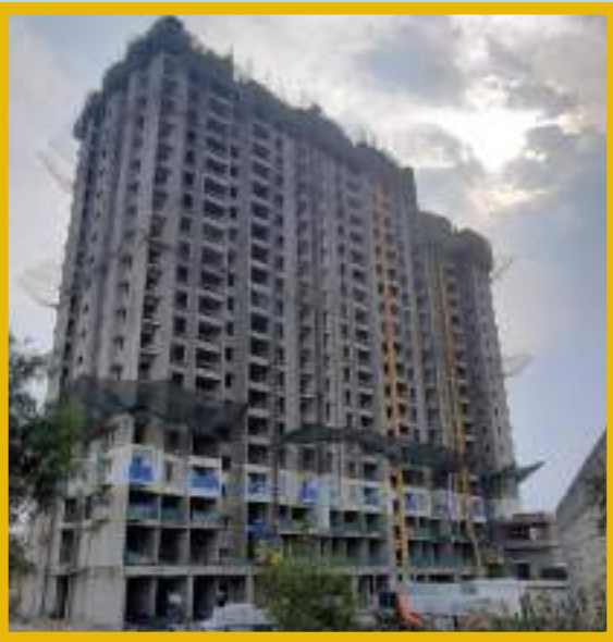
21st floor slab shuttering work is in progress.
