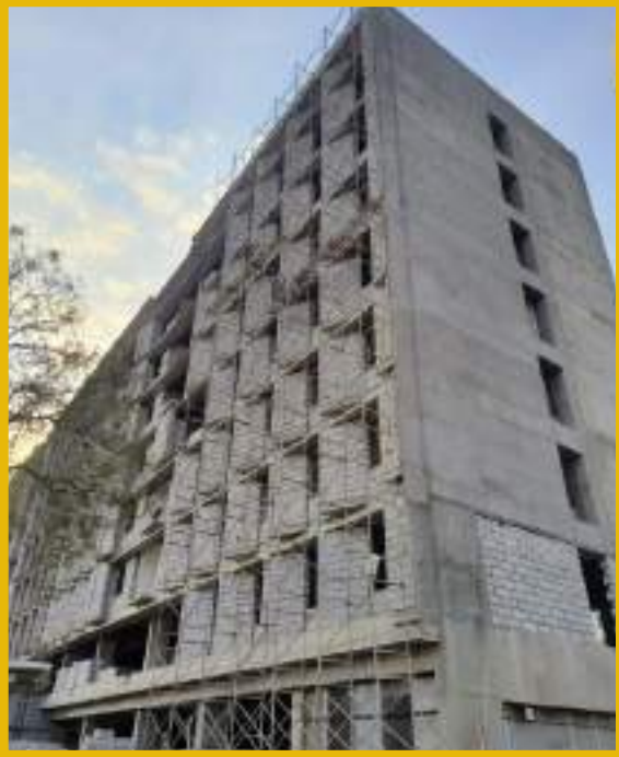
Front side plaster preparation work is in progress.
