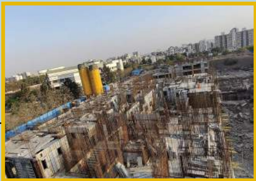
4th slab - Pour 2 Reinforcement binding completed.
