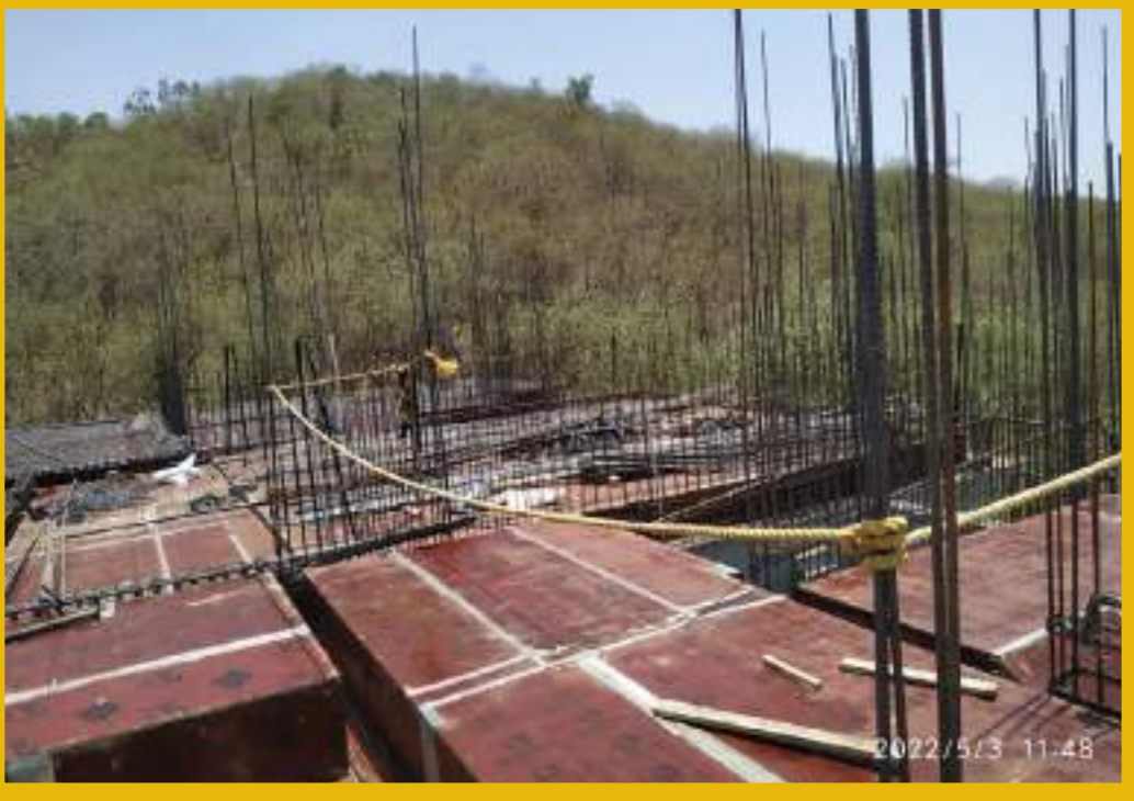
4th floor slab shuttering & steel binding work is in progress.
