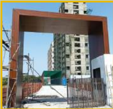
Entrance Gate- ACP cladding work completed.
