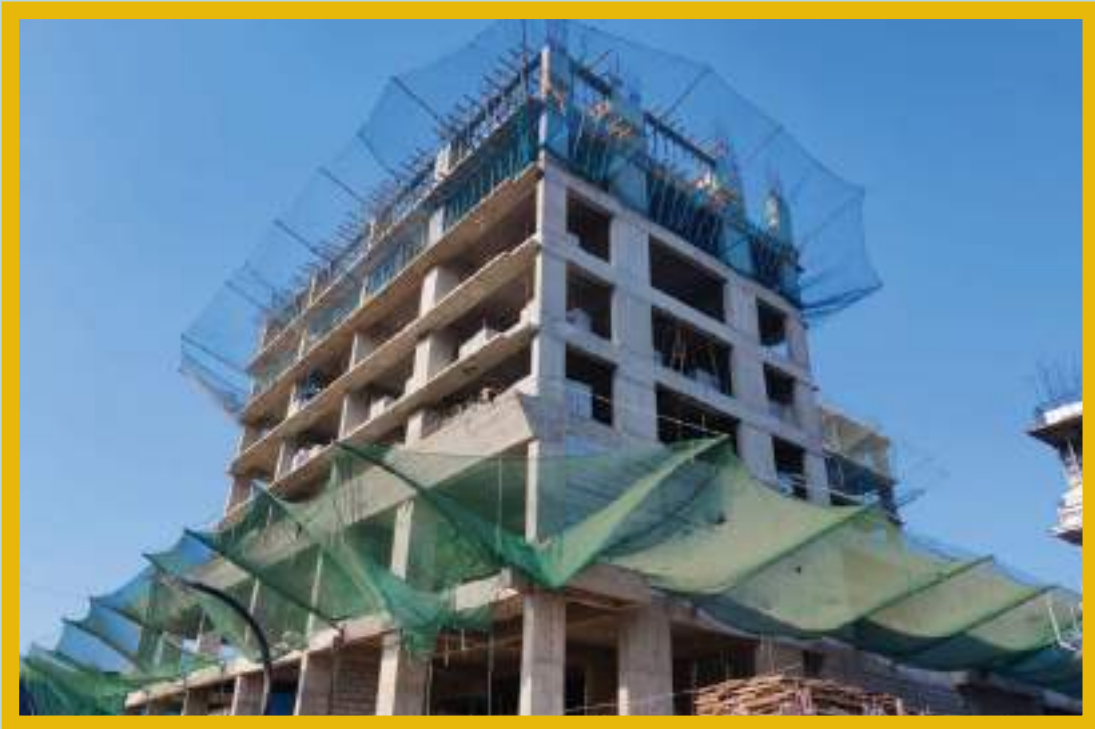
10th slab- Pour 2- Beam Bottom shuttering work is in progress.
