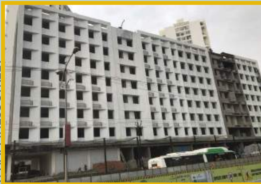
2nd primer paint coat is in progress.
