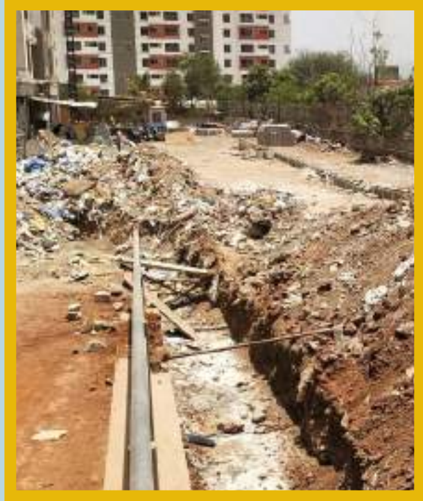
Excavation work for UG services is in progress.
