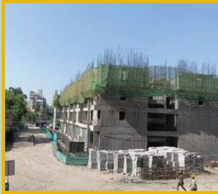
4th floor slab Aluform erection work in progress.
