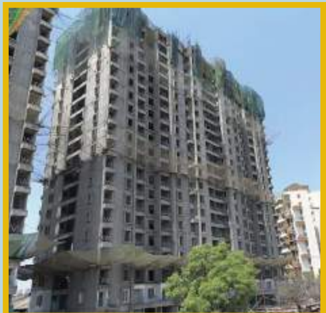
22nd floor slab shuttering and reinforcement work in progress.
