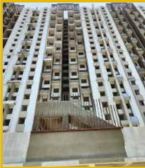
Internal Flat Flooring Work Completed. External Painting. Texture Work 85% Completed.
