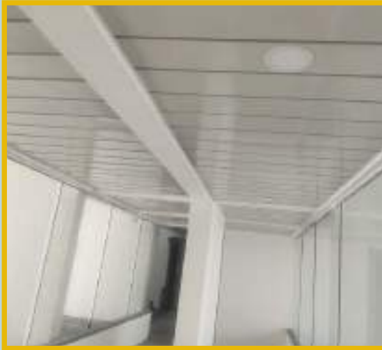
Building A and B - lobby false ceiling work completed.
