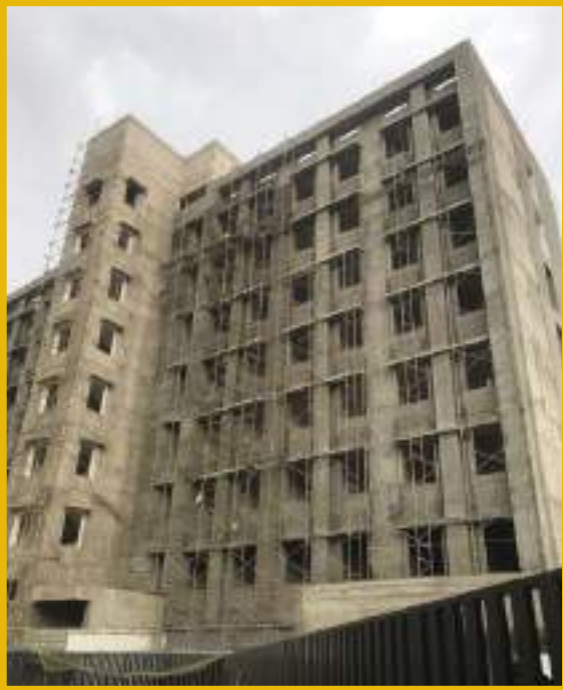
Back side- 2nd coat plaster work is in progress
