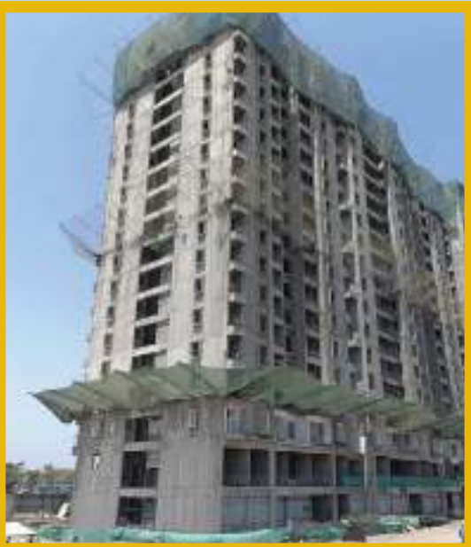
19th floor slab shuttering and reinforcement work in progress.
