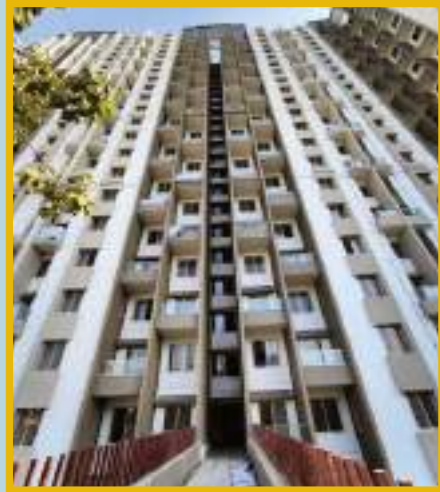
Electrical Mains Wiring & Testing Work In Progress.
