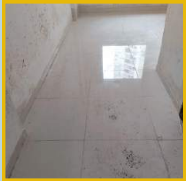
3rd floor tiling is in progress.
