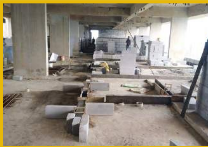
4 th floor blockwork is in progress.
