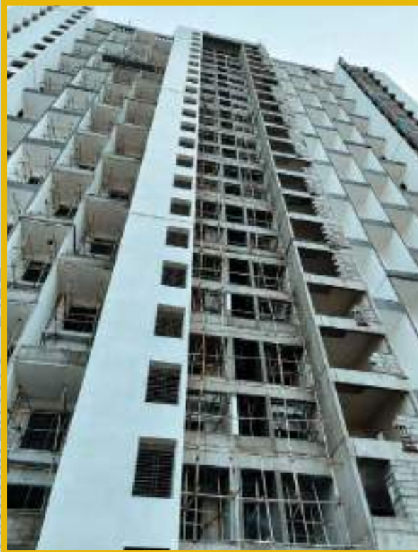
North side external painting work is in progress.
