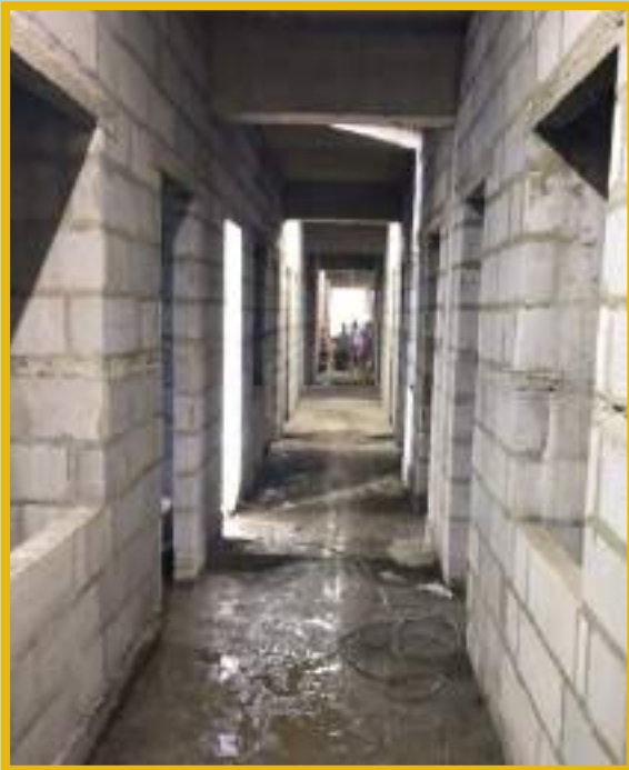
3 rd floor blockwork has been completed.
