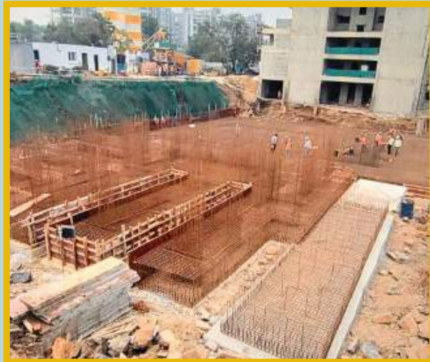
Footing Reinforcement binding work is in progress.
