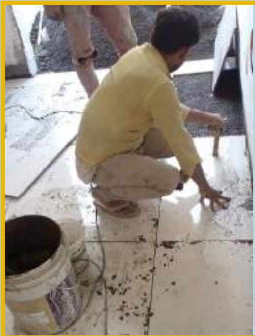
Flooring work is in progress on 16 th floor.
