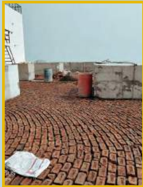
Top terrace brickbat waterproofing work is in progress.
