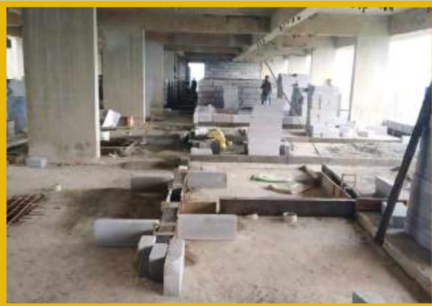
4 th floor blockwork is in progress.
