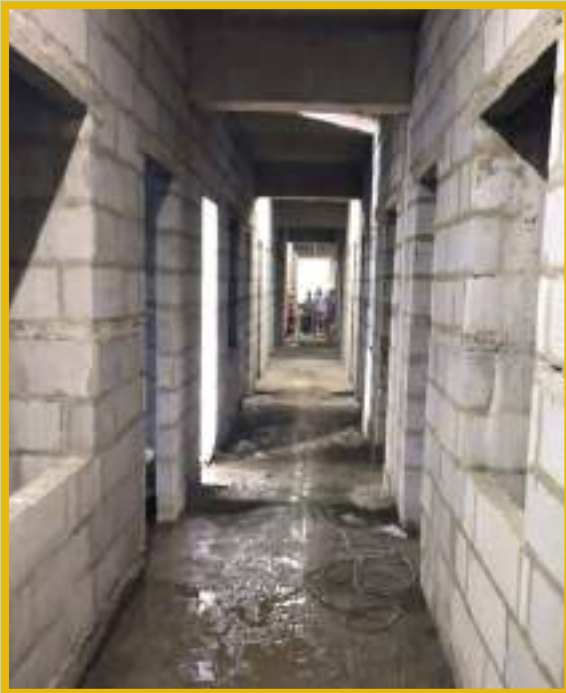
3 rd floor blockwork has been completed.
