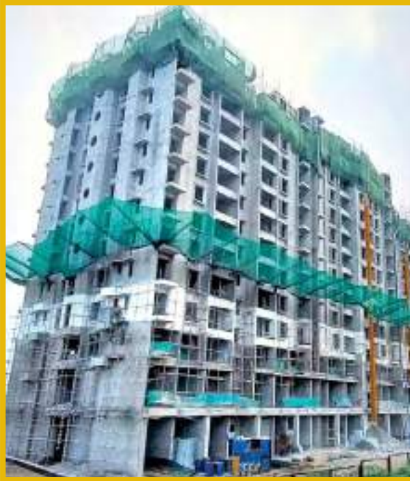
13 th floor slab shuttering work is in progress.
