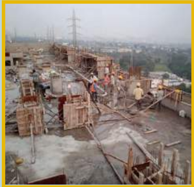
Above terrace duct closing in RCC is in progress.
