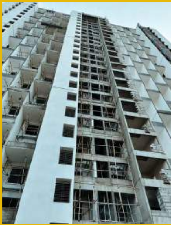
North side external painting work is in progress.
