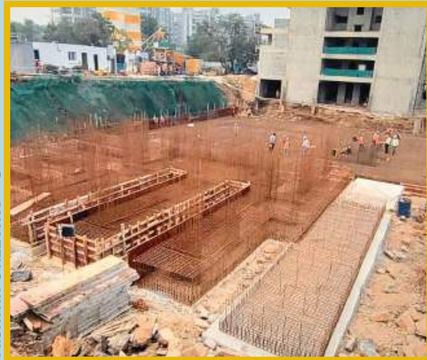
Footing Reinforcement binding work is in progress.
