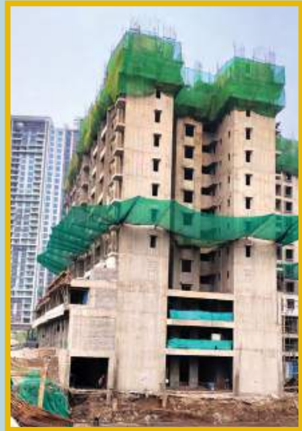
12 th floor slab shuttering work is in progress.
