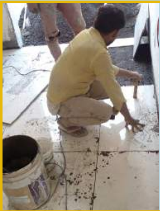
Flooring work is in progress on 16 th floor.
