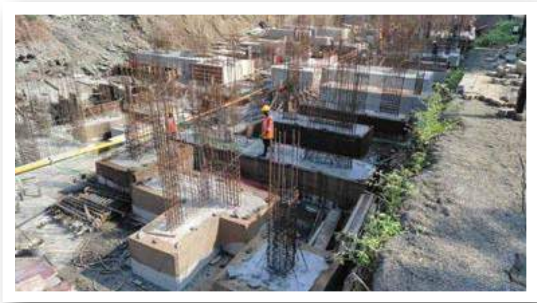
YASHONE ETERNITEE - 'D' FOOTINGS WORK IS IN PROGRESS.
