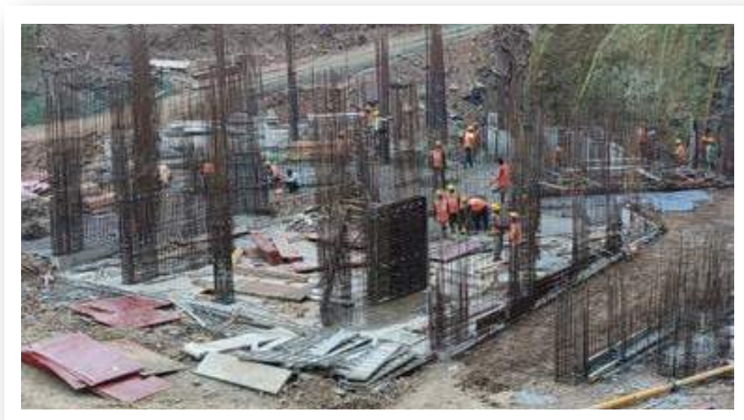
YASHWIN NUOVOCENTRO - 'B' RAFT COMPLETED BY 100%, COLUMN REINFORCEMENT IN PROGRESS.
