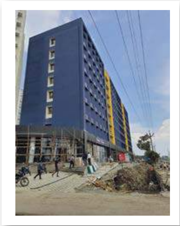
VJ HAPPINESS STREET- LHS FRONT SIDE DEVELOPMENT WORK IS IN PROGRESS.
