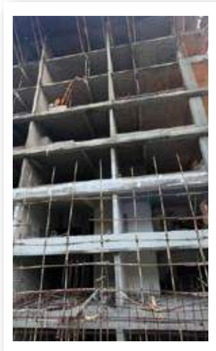
VJ INDILIFE SLAB SHUTTERING & REINFORCEMENT WORK IS IN PROGRESS 10TH FLOOR.
