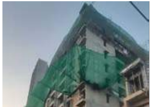
YASHWIN ORIZZONTE - 'D' SLAB WORK IS IN PROGRESS AT 10TH FLOOR.
