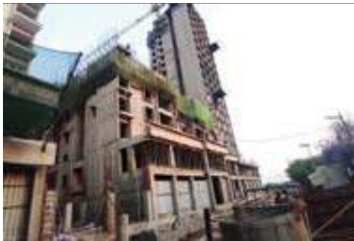
YASHWIN ORIZZONTE - 'C' SLAB WORK IS IN PROGRESS AT 6TH FLOOR.
