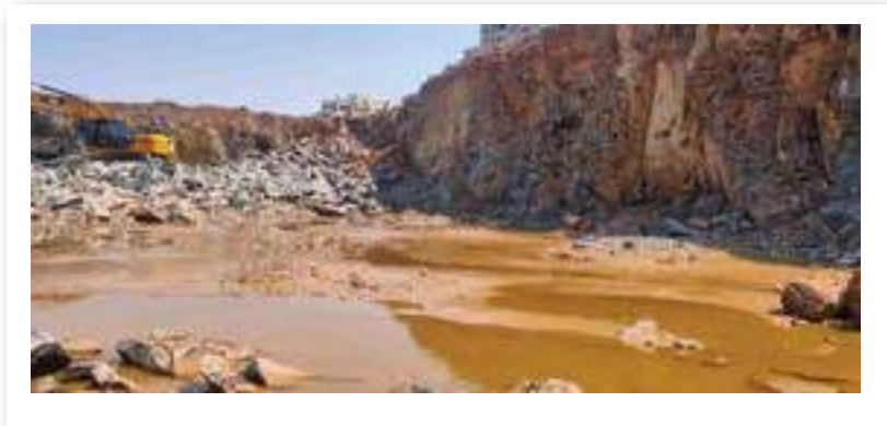
YASHWIN ENCHANTÉ - 'B1-B2' EXCAVATION WORK IS IN PROGRESS.
