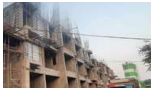
YASHWIN ORIZZONTE - 'E' SLAB WORK OF MOCK FLOOR IS IN PROGRESS.
