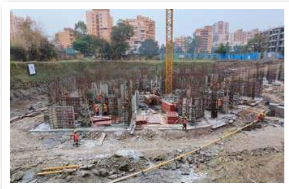
YASHWIN NUOVOCENTRO - 'A' 80% COLUMNS COMPLETED IN BASEMENT 2 LEVEL.
