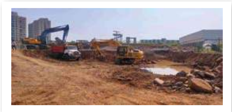
YASHWIN ENCHANTÉ - 'D1-D2' SOFT MURUM REMOVING WORK IS IN PROGRESS.
