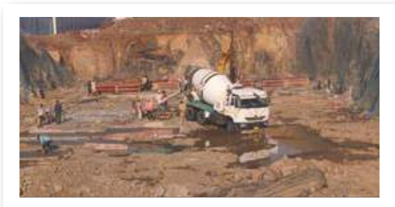
YASHWIN ENCHANTÉ - 'F1-F2' FOOTING PCC WORK IS IN PROGRESS.
