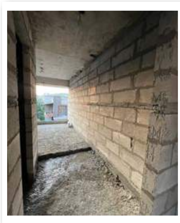
VJ INDILIFE AAC BLOCKWORK IS IN PROGRESS AT 4TH FLOOR.
