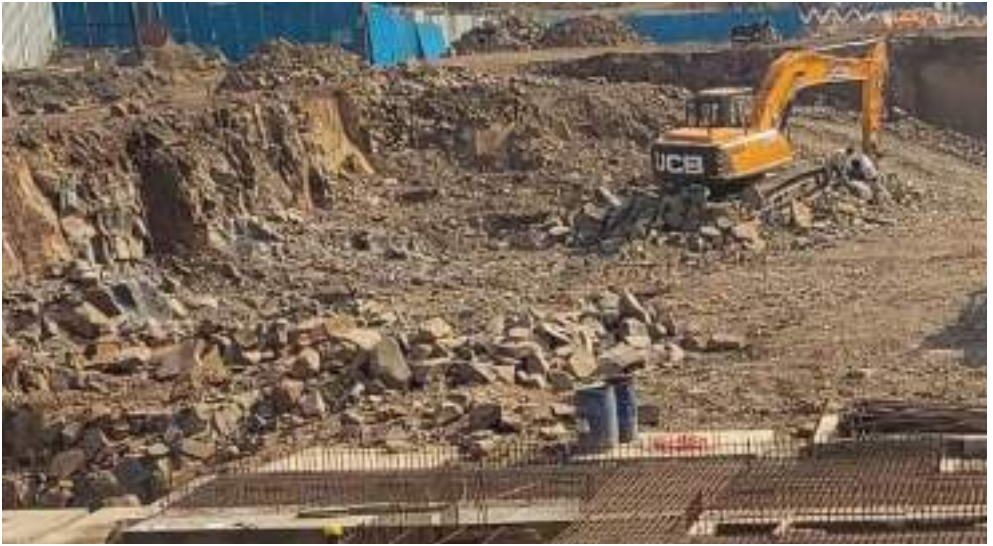
Yashwin Orizzonte 'D' - Excavation work is in progress.
