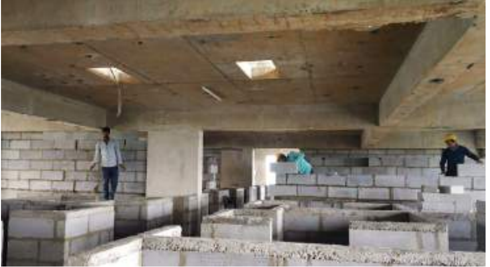
VJ HAPPINESS STREET - 3 rd floor blockwork is in progress.
