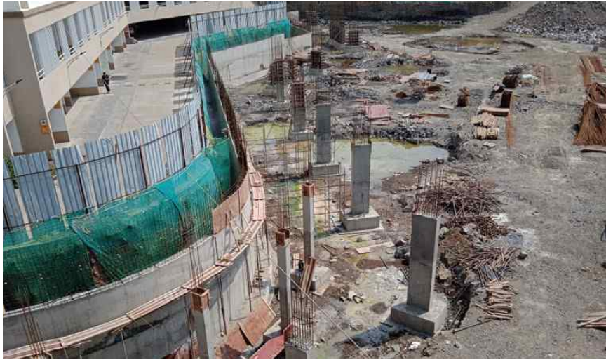
VJ HAPPINESS STREET - RHS - COLUMN & RETAINING WALL WORK HAS BEEN COMPLETED.
