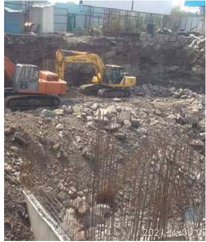
YASHWIN ENCORE - COMMERCIAL BUILDING EAST SIDE EXCAVATION WORK IS IN PROGRESS.
