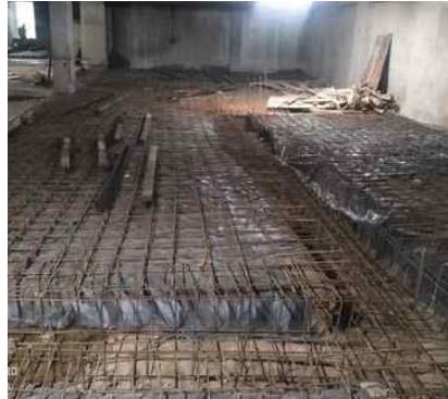
YASHWIN ENCORE - CENTRAL PODIUM - BASEMENT RAFT REINFORCEMENT WORK IS IN PROGRESS.
