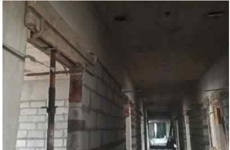
YH-RYAN SCHOOL- LINTEL CASTING WORK IS IN PROGRESS ON 4 TH FLOOR.
