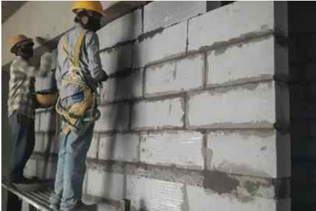
YH-RYAN SCHOOL- BLOCKWORK IS IN PROGRESS ON 5 TH FLOOR.
