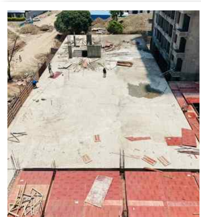
YASHONE MAAN-HINJAWADI - MULTIPURPOSE HALL- PARAPET & LMR SHUTTERING WORK IS IN PROGRESS.
