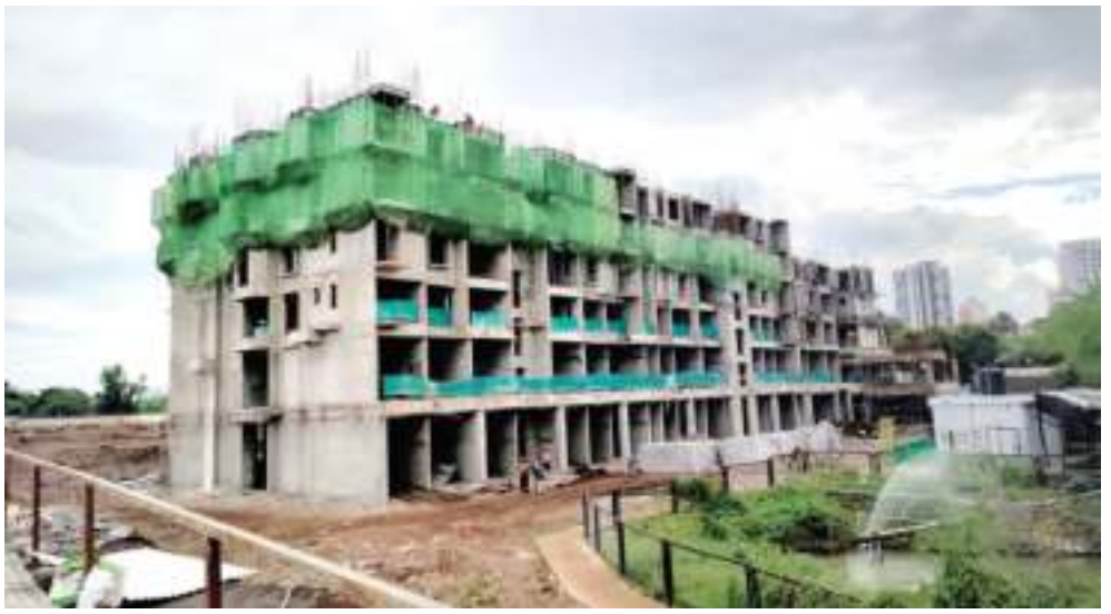
Yashwin Orizzonte 'A' - 5 th floor slab work is in progress.
