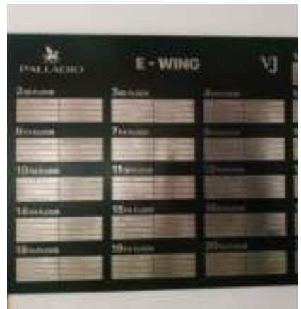
PALLADIO 'E'- Name board fixing work has been completed.
