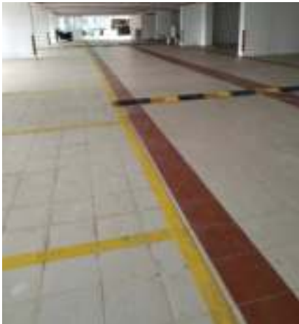
PALLADIO 'E' - Lower & upper parking tiles grouting work is in progress.
