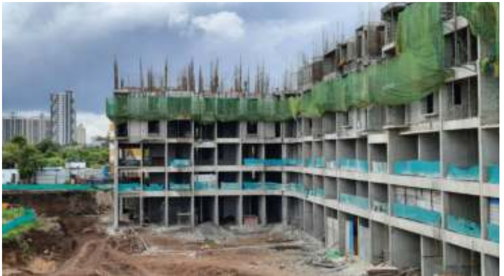
Yashwin Orizzonte 'B' - 4 th floor slab shuttering work is in progress.
