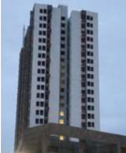
Yashwin Encore 'B1B2' - West side external painting work is in progress.
