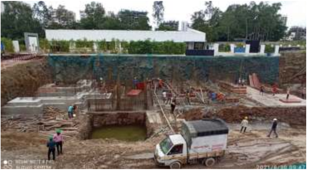
Yashwin Supernova 'C' - Footing casting work is in progress.
