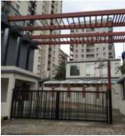
PALLADIO 'E' - Entrance gate painting work has been completed.
