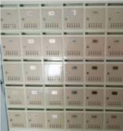
PALLADIO 'E'- Letter box fixing work has been completed.
