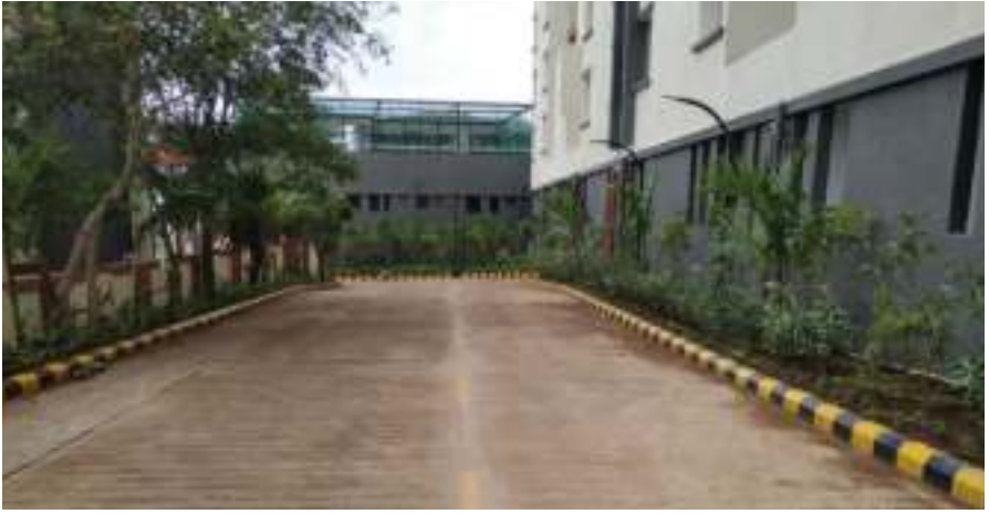
PALLADIO 'E'- Entrance gate plantation & kerb stone fixing work has been completed.
