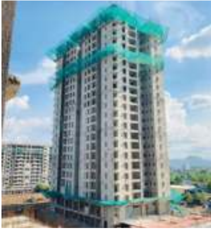
YashONE Hinjawadi - PODIUM PH -1- Shuttering work is in progress for sitouts, trimix concrete work is in progress in lower parking.
