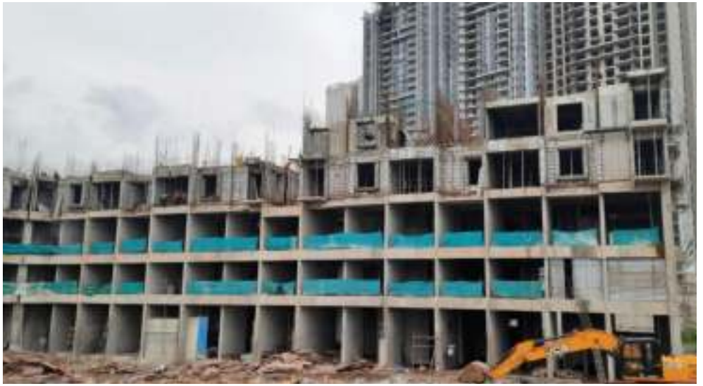
Yashwin Orizzonte 'A' - 3 rd floor slab shuttering work is in progress.
