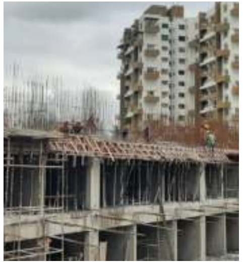
YashONE Infinitee 'D1D2' - 2 nd floor slab aluminium shuttering mock-up work is in progress. 1 st floor slab casting has been completed.
