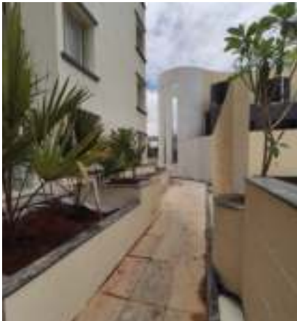
PALLADIO 'E' - Podium texture work is in progress.
