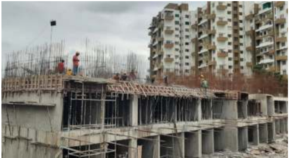
YashONE Infinitee 'D1D2' - 2 nd floor slab aluminium shuttering mock-up work is in progress. 1 st floor slab casting has been completed.
