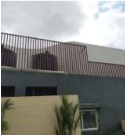
PALLADIO 'E' - Railing fixing above multi-purpose hall is completed.
