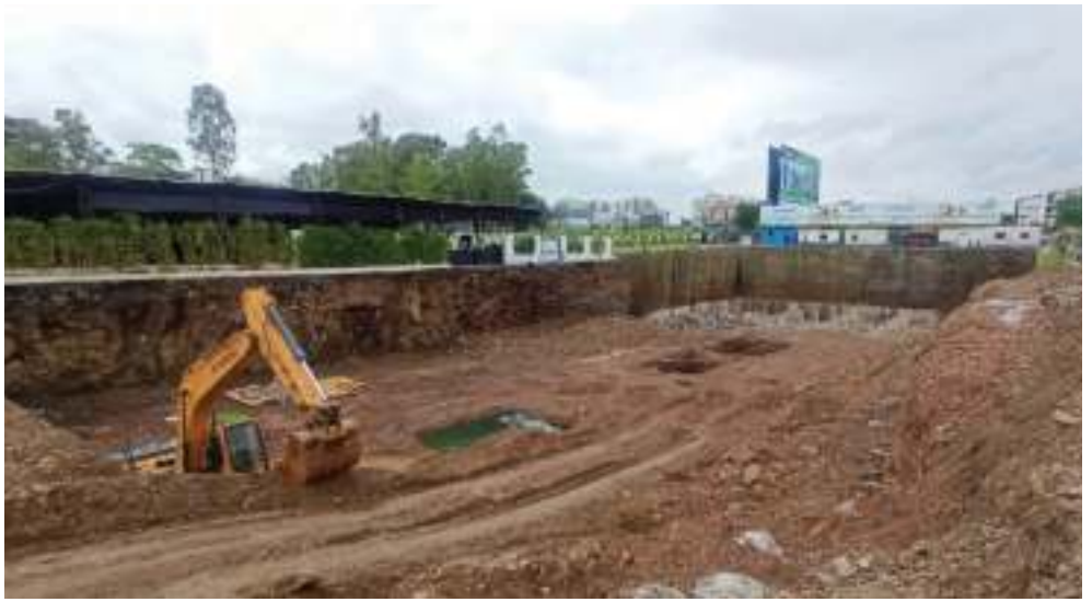
Yashwin Supernova 'C' - Excavation work has been completed.
