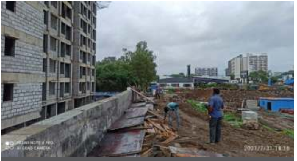
Yashwin Supernova - West side retaining (plum) wall work is in progress.
