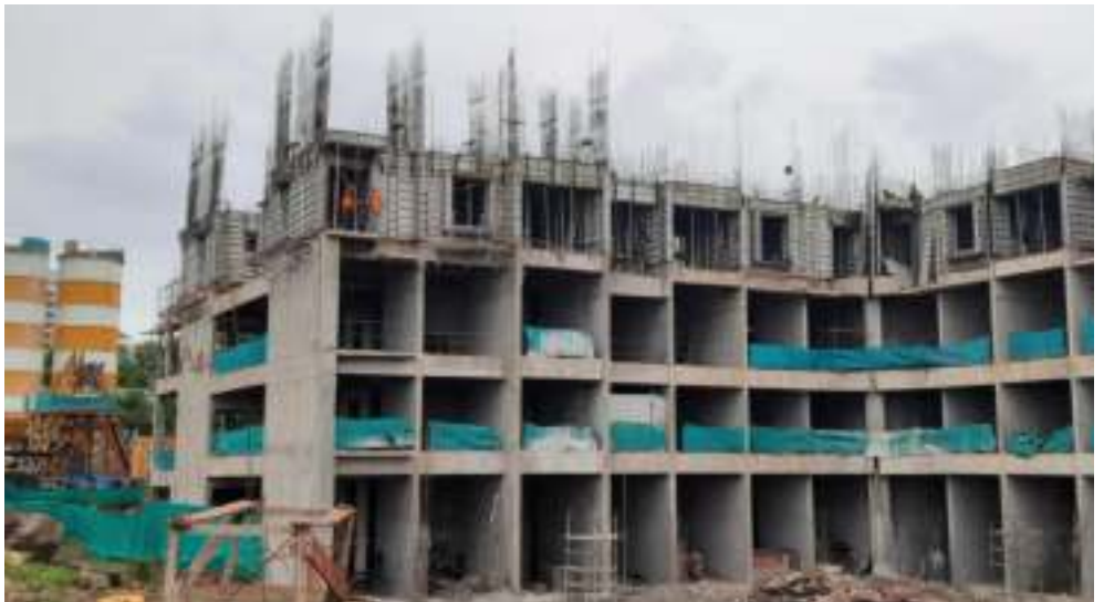
Yashwin Orizzonte 'B' - 3 rd floor slab shuttering work is in progress.
