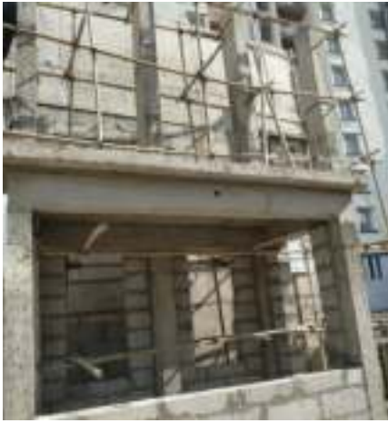
PALLADIO 'E' - Entrance gate side wall ACP work is in progress.
