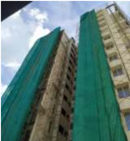
PALLADIO 'E' - West side external plaster work is in progress.
