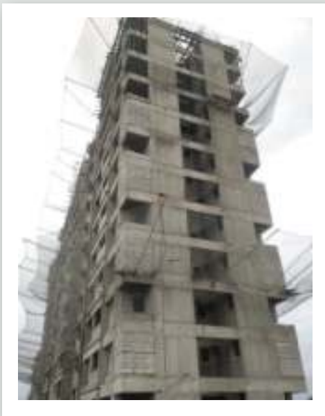
Yashwin Sukhniwas 'B' - 12 th floor shearwall work is in progress, blockwork has been completed till 8 th floor.
