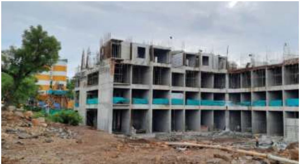
Yashwin Orizzonte 'B' - 4 th slab shuttering work is in progress.
