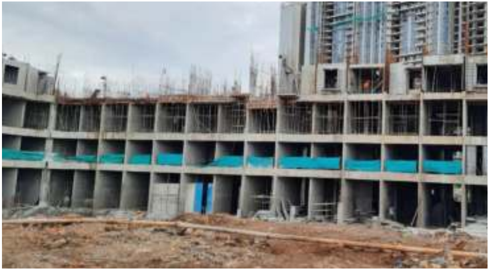
Yashwin Orizzonte 'A' - 4 th slab shuttering work is in progress.
