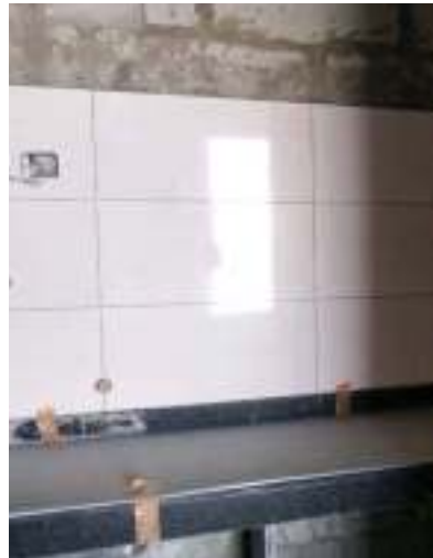
PALLADIO - P2 - KITCHEN DADO TILE WORK COMPLETED UPTO 14 TH FLOOR.
