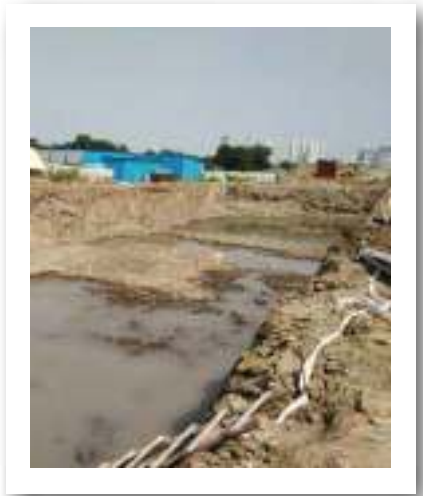
YASHWIN SUKHWI WAS - 'C' - 3. YSNW - C EXCAVATION WORK HAS BEEN COMPLETED.
