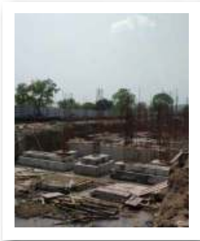
YASHWIN SUKHWI WAS - 'B' - FOOTING CASTING COMPLETED. SHEARWALL AND REINFORCEMENT AND SHUTTERING WORK IS IN PROGRESS.
