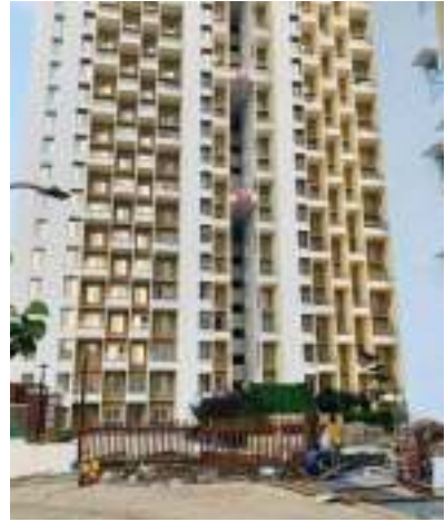
YASHWIN HINJAWADI - 'B' - PODIUM ENTRY GATE FABRICATION WORK COMPLETED.
