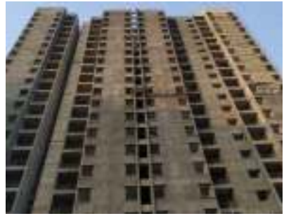
PALLADIO - P2 - E - SOUTH SIDE EXTERNAL PLASTER WORK IS IN PROGRESS.
