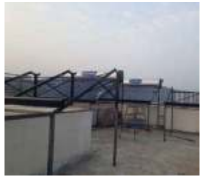
YASHWIN HINJAWADI - 'B' SOLAR TUBE & PANEL FIXING WORK IS IN PROGRESS.
