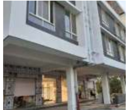
YASH 101 - EXTERNAL PAINTING WORK IS IN PROGRESS.
