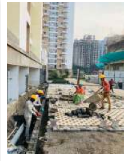
YASHWIN HINJAWADI - 'B' PAVER BLOCK & GRASS PAVER FIXING WORK AT EAST SIDE OF B BUILDING WORK IS IN PROGRESS.
