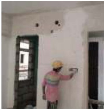
PALLADIO - P2 - GYPSUM WORK IS IN PROGRESS ON 19 TH & 20 TH FLOOR.
