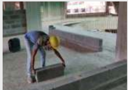
RYAN SCHOOL - A BLOCK BLOCKWORK LINEOUT WORK IS IN PROGRESS.
