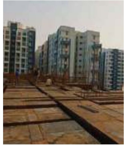
YASH 101 - 6 TH FLOOR SLAB WORK IS IN PROGRESS.
