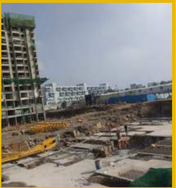
Footing steel binding work is in progress.
