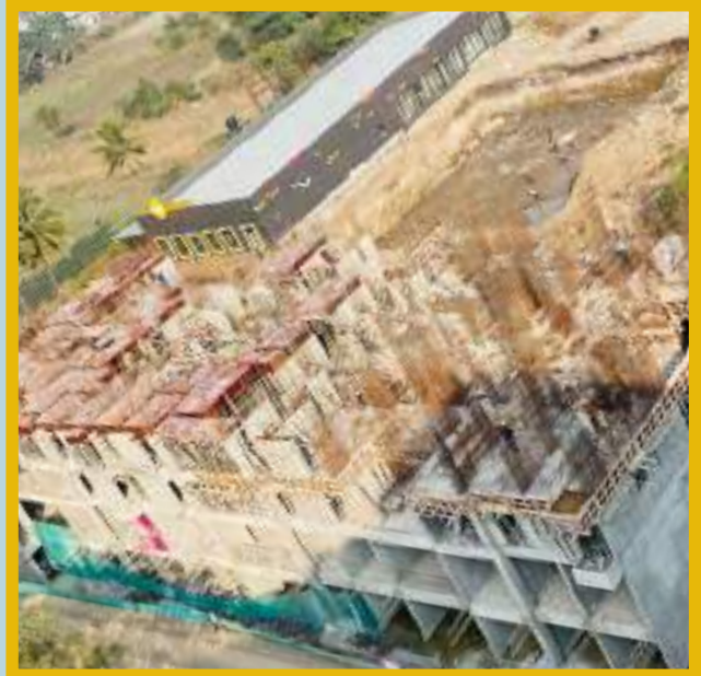
3rd floor Slab shuttering and Reinforcement work is in progress.
