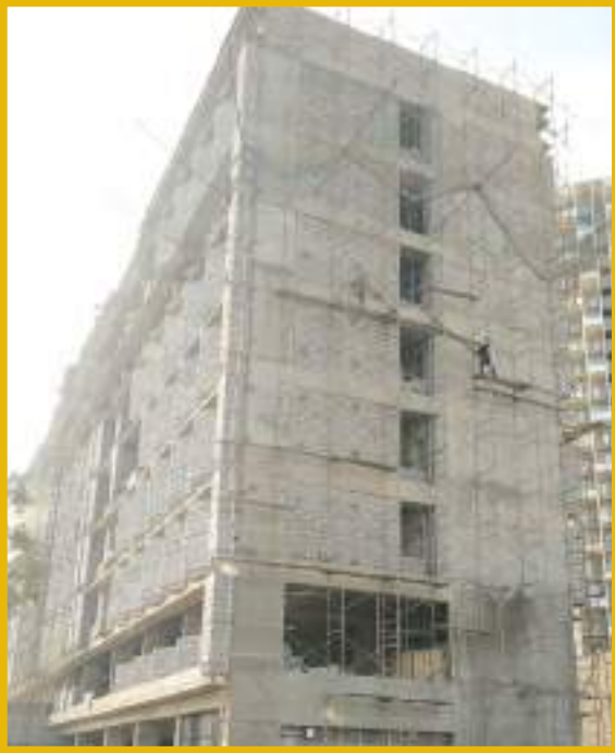
External plaster preparation is in progress.
