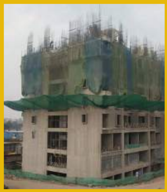
8th floor Slab Shuttering and Reinforcement work is in progress.
