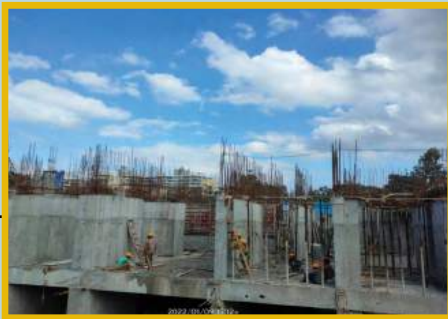
2nd Slab- Pour 2 slab decking work is in progress.
