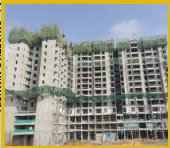
15th floor slab shuttering work is in progress.
