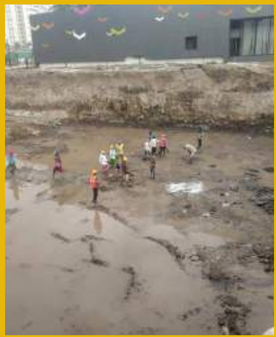
Surface Preparation for PCC work.
