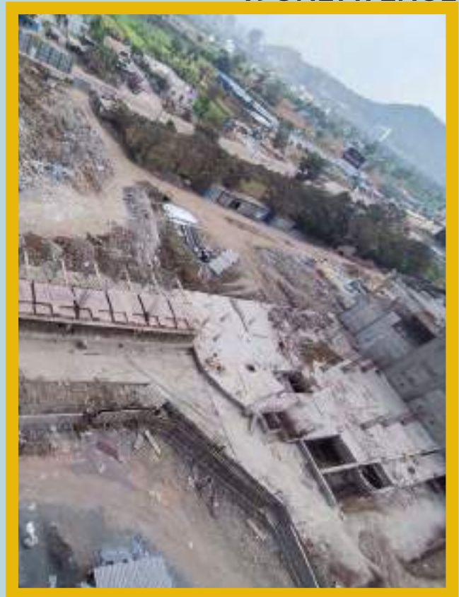
RHS side- Y block- 1st Slab 100% completed.
