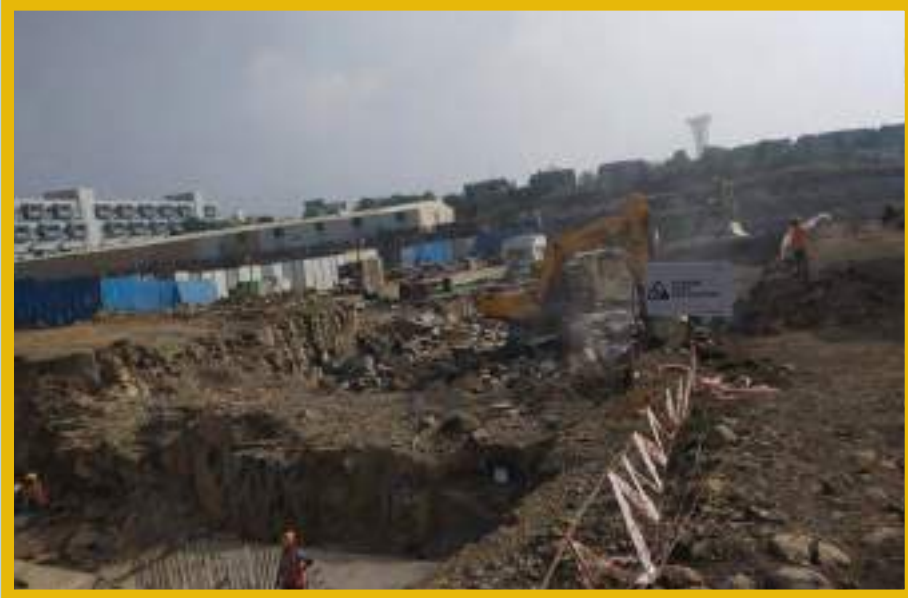
Excavation work is in progress.
