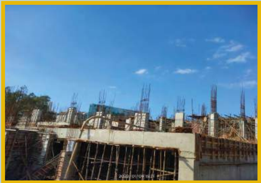
4th slab- Pour 2 above 3rd slab column casting work is in progress.
