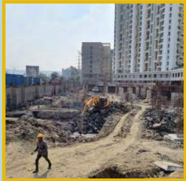
Excavation, Footing, Column and Retaining wall work is in progress.
