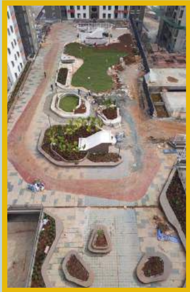
Plantation work is in progress.
