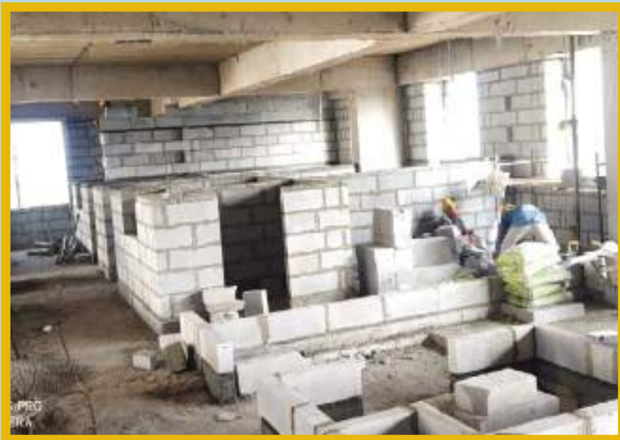
7th floor Block Work is in progress.
