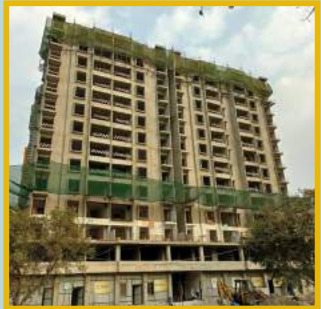
15th floor slab shuttering work is in progress.
