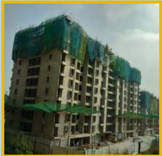
11th floor slab casting 50% done. 12th floor slab shear wall reinforcement work is in progress.
