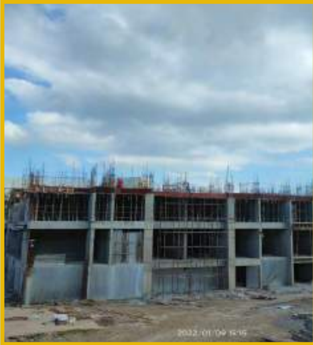
3rd Slab- Pour 1 slab reinforcement work is in progress.
