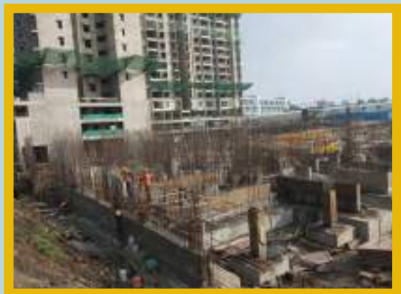
Stub column upto plinth- casting work is in progress.
