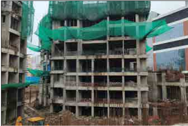
YASHWIN NUOVOCENTRO - 'B' RCC WORK IS IN PROGRESS AT 6TH FLOOR.
