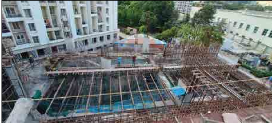
VJ HAPPINESS STREET-RHS 5TH SLAB - SHUTTERING WORK IS IN PROGRESS.
