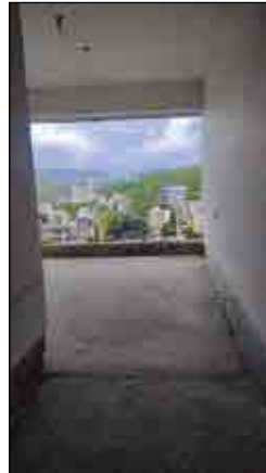
VJ INDILIFE INTERNAL GYPSUM WORK IS IN PROGRESS AT 14TH FLOOR.
