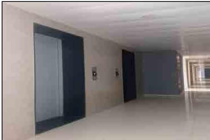
VJ GRAND CENTRAL LIFT INSTALLATION WORK IS IN PROGRESS.
