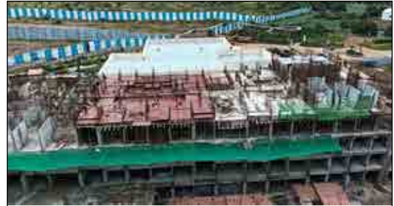
YASHWIN ENCHANTÉ - 'D1+D2' SLAB CASTING WORK IS 40% COMPLETED AT 2ND FLOOR.
