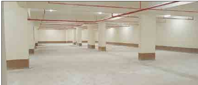
VJ TOWN CENTRE Basement 1&2 parking first coat painting work is completed.
