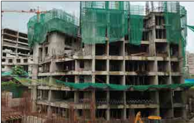
YASHWIN NUOVOCENTRO - 'A' RCC WORK IS IN PROGRESS 5TH FLOOR.
