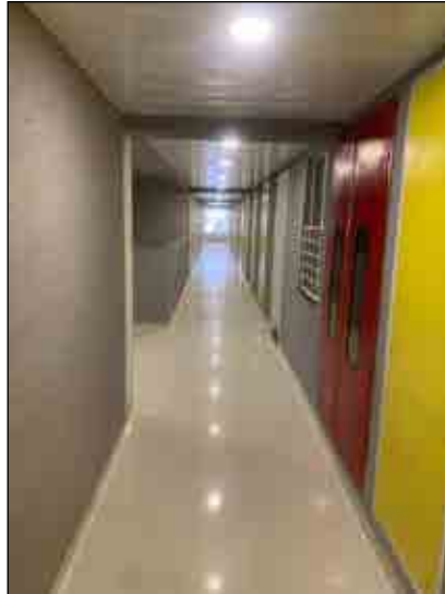
VJ TOWN CENTRE Basic cleaning work is completed till 12th floor.
