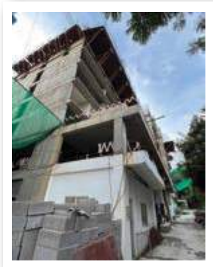
VJ INDILIFE 7TH FLOOR 2ND POUR SHUTTERING & STEELWORK IS IN PROGRESS.
