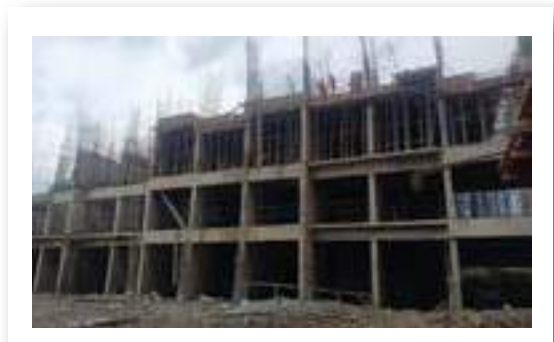
YASHWIN ORIZZONTE - 'E' 2ND FLOOR SLAB SHUTTERING WORK IS IN PROGRESS.
