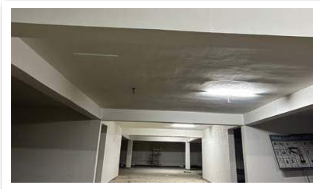
VJ INDILIFE BASEMENT FINE PUTTY WORK IS IN PROGRESS..
