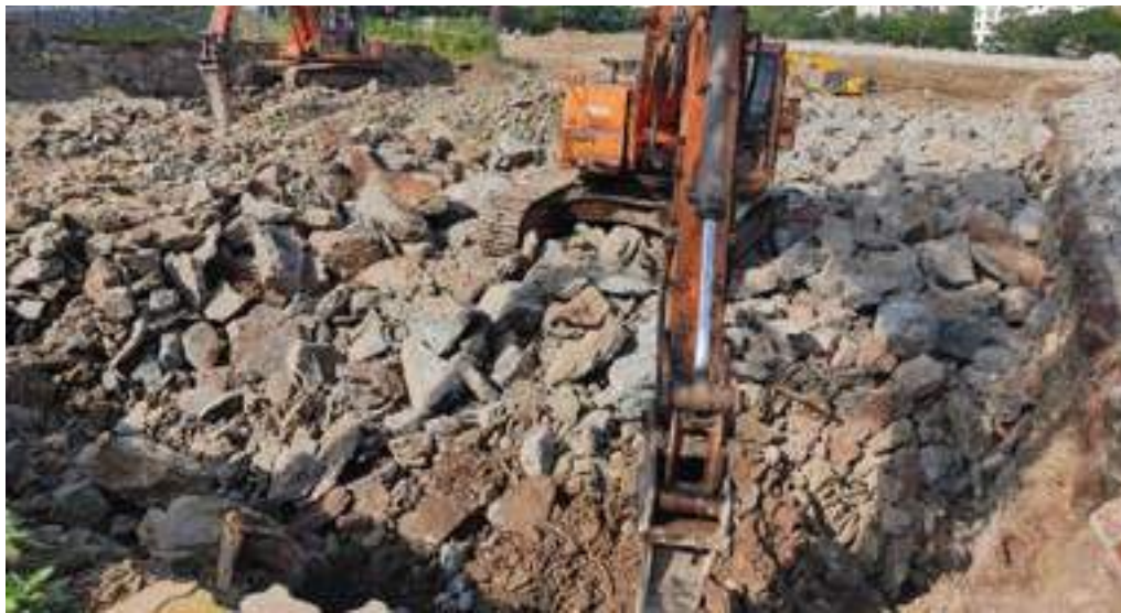
YASHWIN ETERNITEE - 'D' EXCAVATION IN HARD STRATA IS IN PROGRESS.
