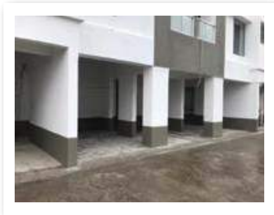
YASHWIN SUKHNIWAS - 'D' PARKING FLOORING WORK IS IN PROGRESS.
