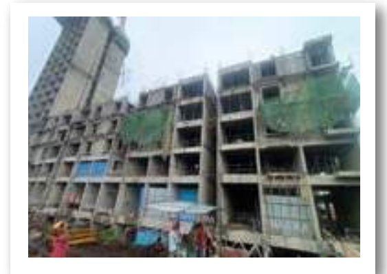
YASHWIN ORIZZONTE - 'D' 5TH FLOOR SLAB SHUTTERING WORK IS IN PROGRESS.
