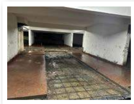
VJ INDILIFE BASEMENT TREMIX WORK IS IN PROGRESS.
