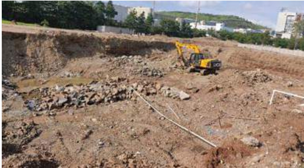
YASHWIN ETERNITEE - 'C' LIFT PIT EXCAVATION WORK IS IN PROGRESS.
