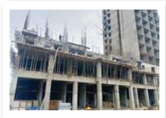
YASHWIN ORIZZONTE - 'C' 4TH FLOOR SLAB SHUTTERING WORK IS IN PROGRESS.
