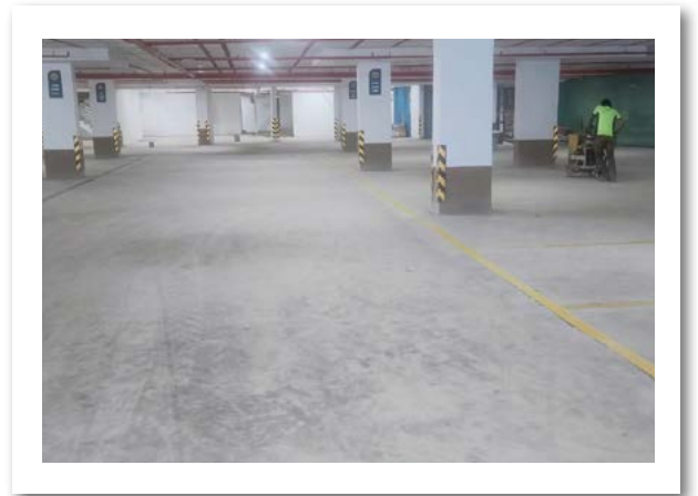
YASHONE HINJAWADI - 'D' LOWER PARKING THERMOPLASTIC PAINTING WORK IS IN PROGRESS FOR CAR PARKING.
