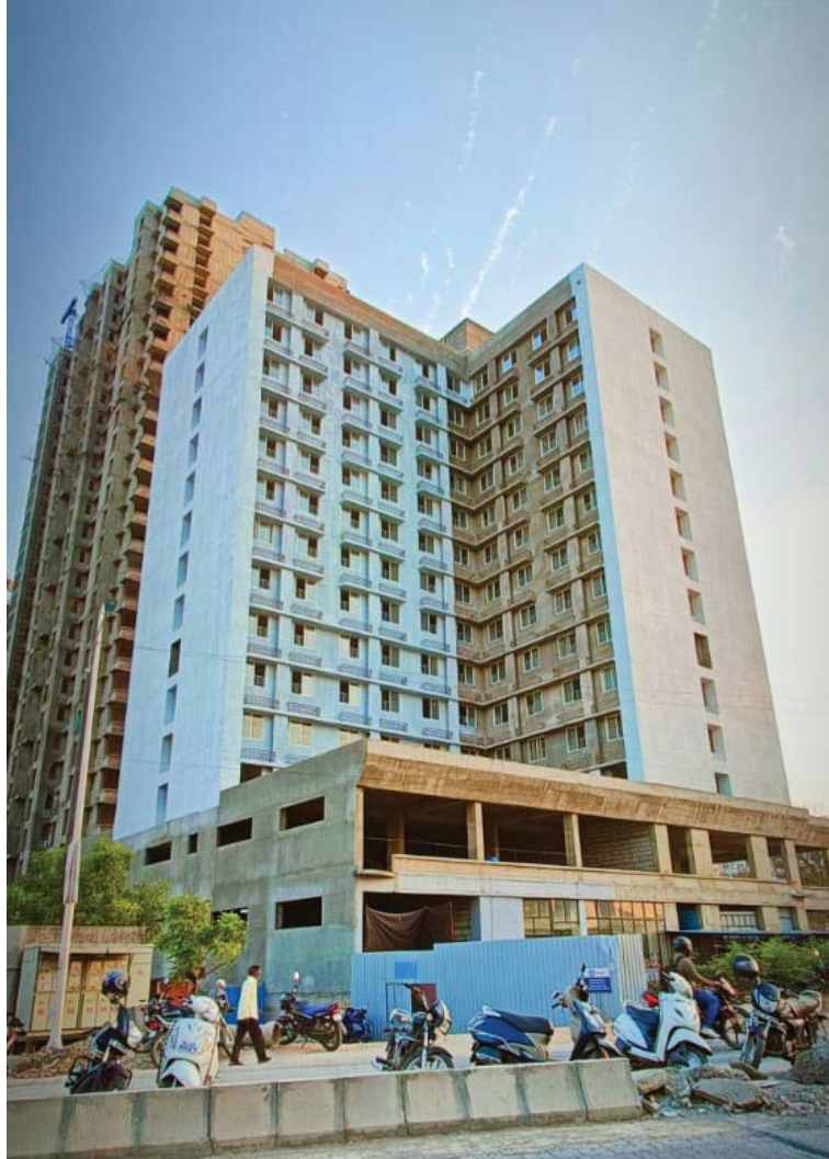
VJ TOWN CENTRE EXTERNAL PAINTING - PRIMER WORK IS IN PROGRESS.
