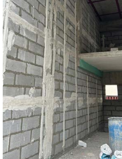
VJ HAPPINESS STREET - RHS GF SHOPS GYPSUM WORK IS IN PROGRESS.
