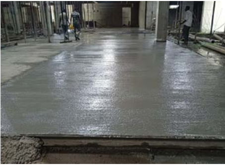
VJ HAPPINESS STREET - RHS BASEMENT TREMIX WORK IS IN PROGRESS.
