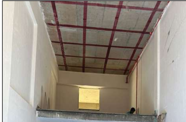
VJ HAPPINESS STREET- RHS GF SHOPS FLOORING WORK IS IN PROGRESS.
