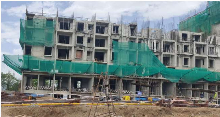
YASHONE ETERNITEE - 'C' 4TH FLOOR SLAB CASTING IS COMPLETED.
