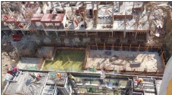
YASHWIN ENCHANTÉ - UGWT WALL REINFORCEMENT WORK IS COMPLETED.
