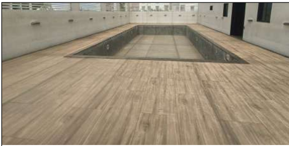
YASHONE HINJAWADI - SWIMMING POOL LINER WORK IS IN PROGRESS.
