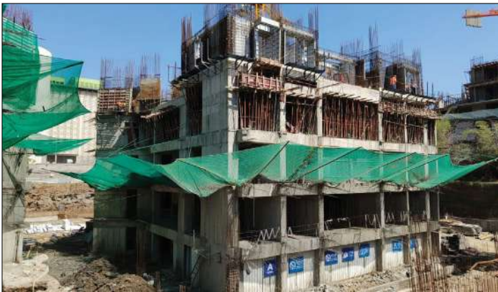
YASHWIN NUOVOCENTRO - 'A' 2ND FLOOR RCC WORK IS IN PROGRESS.
