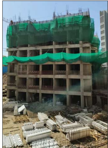
YASHWIN NUOVOCENTRO - 'B' 3rd floor RCC work is in progress.
