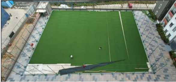
YASHONE HINJAWADI - MULTI PURPOSE COURT TURF FIXING WORK IS IN PROGRESS.
