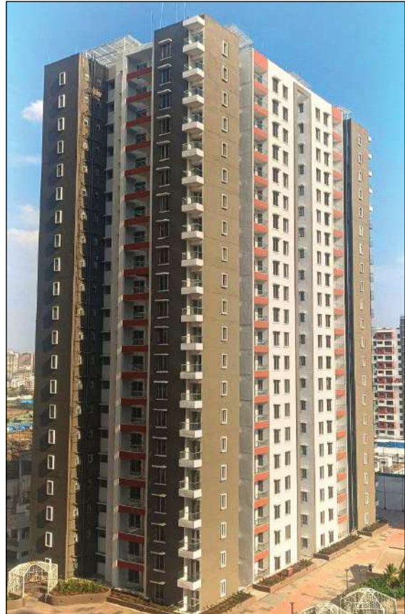
YASHONE HINJAWADI - 'D' 3 LIFTS HANDED OVER. POSSESSION FOR D BUILDING STARTED.
